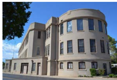
Top: Hill Street school prior to remodelling
